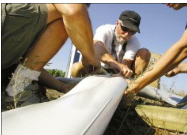
Western Michigan University professor John Patten, center, attaches blades to a wind turbine, on which he spent more than $10,000 of his own money, in preparation for its installation at WMU’s College of Engineering and Applied Sciences.
