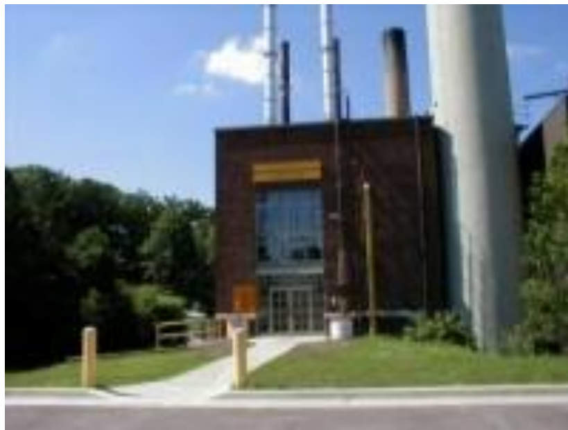
Robert M. Beam Power Plant
