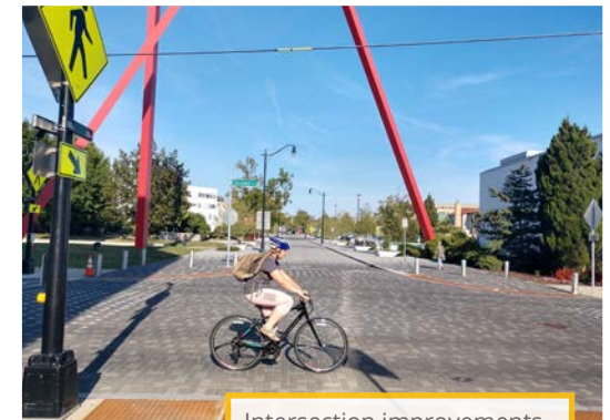
Intersection improvements such as raised crossings and use of varied textures can enhance both accessibility and safety.
