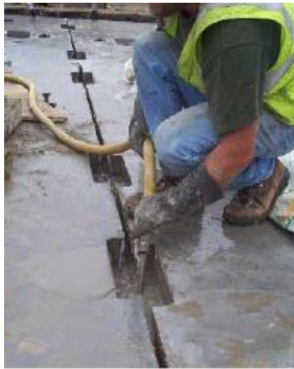
Figure 2-7. Pumping W.R. Meadows Sealight CG-86 non-shrink grout (Source: Oliva et al. 2007)
