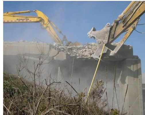
Figure 5-62. Demolition by hammer and pulverizer
