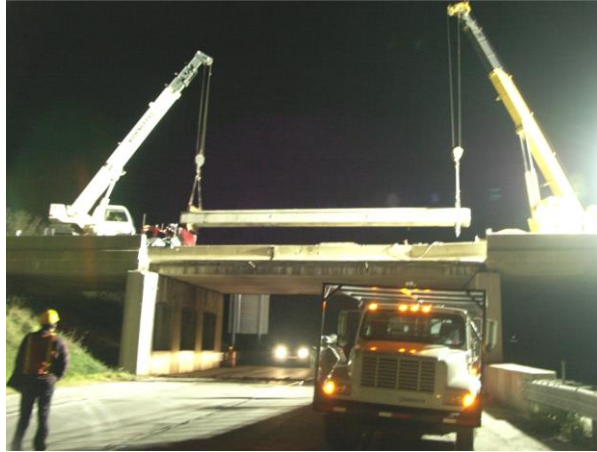
Figure 5-63. Removal of a box-beam
