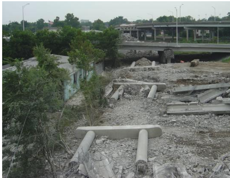
Figure 5-67. Demolition of a bent cap and columns as a single unit (Source: SCDOT)
