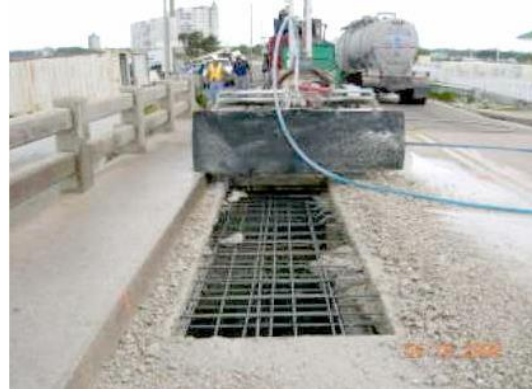
Figure 5-60. Saw cutting technique
