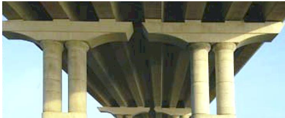
Figure 5-21. Trapezoidal bent cap (Source: Restrepo et al. 2011)
