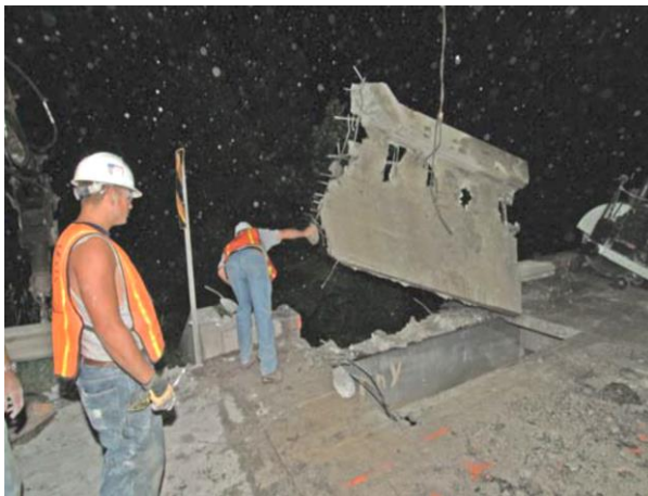
(a) Lifting of a deck panel
