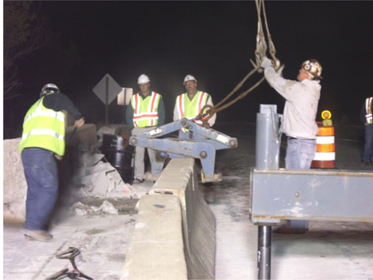
Figure 5-65. Removal of safety barriers
