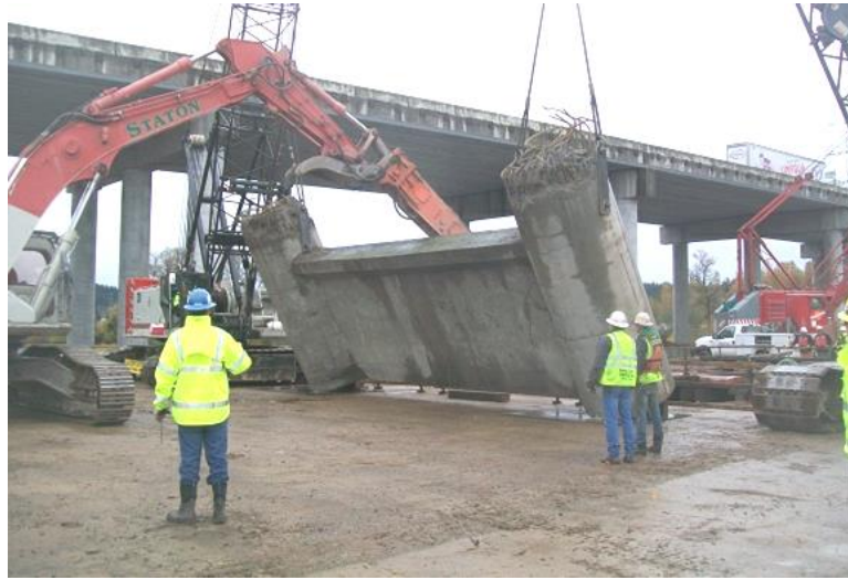
Figure 5-68. Column and pier walls are sawn off and lifted out for demolition (Source: http://www.mcgee-engineering.com )
