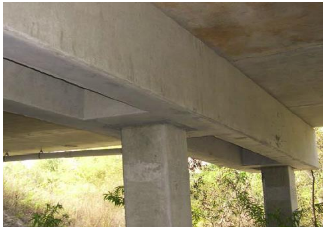
Figure 5-24. Precast bent cap with cavities (Source: Culmo 2009)
