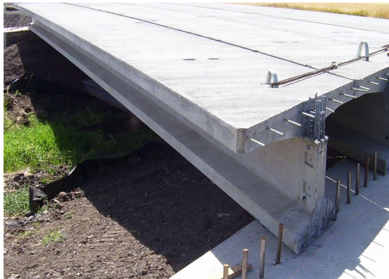
Figure 5-6. Decked bulb-tee girder (Source: CPMP 2011)
