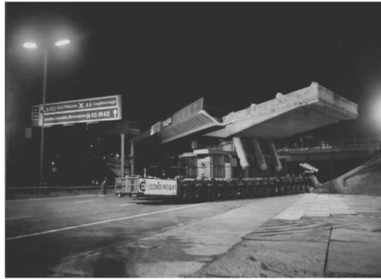
Figure 2–10. Transportation of the Warren Farm Bridge (Source: Anumba et al. 2003)
