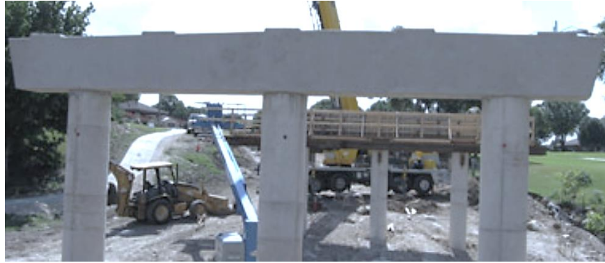
Figure 5-20. Rectangular bent cap (Source: http://facilities.georgetown.org/2009 )
