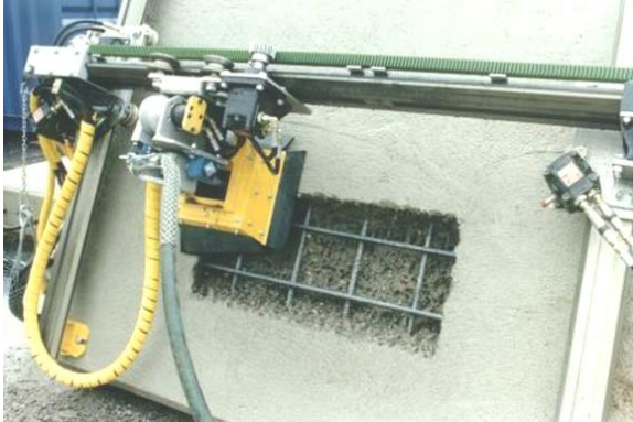
Figure 5-60. Saw cutting technique
