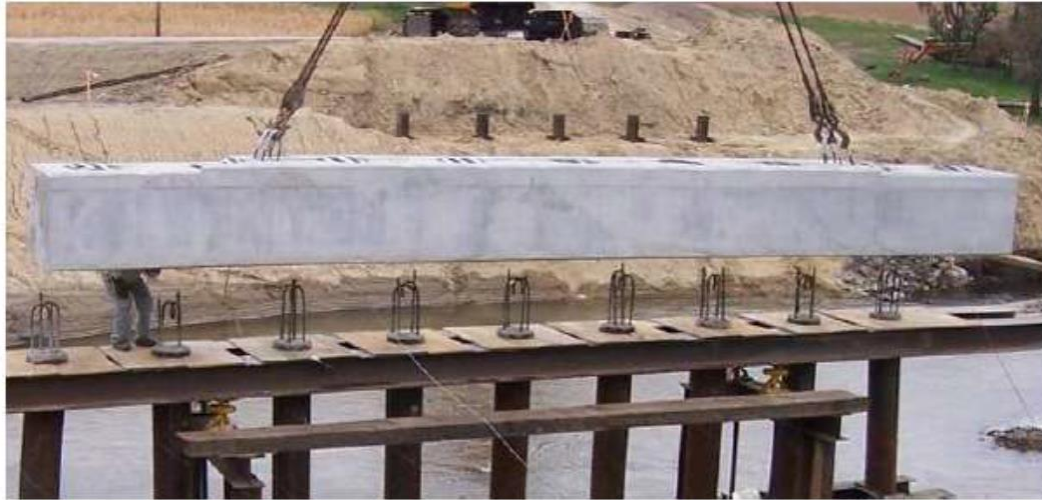
Figure 5-43. Temporary support system for pile cap to pile connection (Source: Wipf et al. 2009a)
