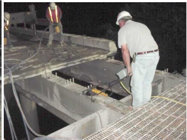
(b) Cutting off the existing steel shear studs
