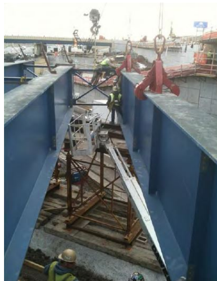
Figure 2-28. Steel I-girder being lifted using beam clamps (FHWA 2015)
