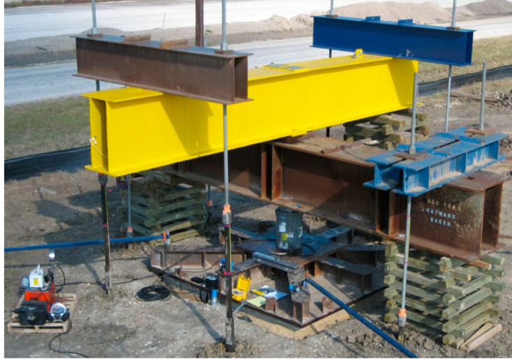
Figure 2-13. Reaction frame and loading setup for a footing (Stuedlein and Holtz 2012)
