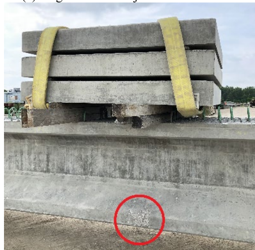
(b) A close-up view of the bottom flange honeycomb
