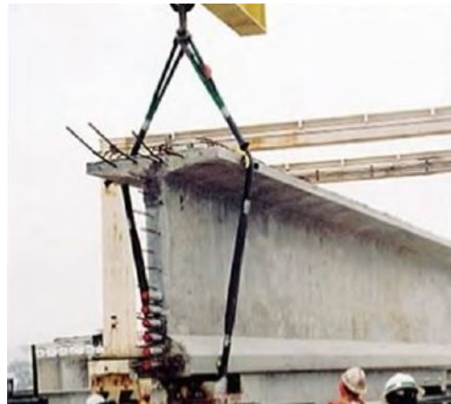
(b) PC girder being lifted using basket hitch
