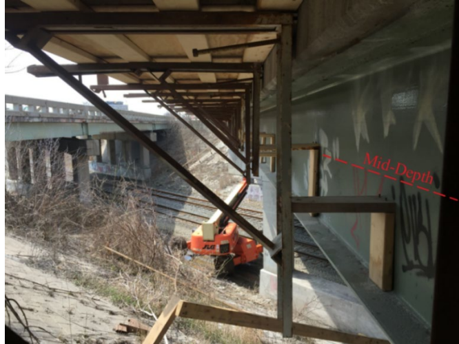
Figure 2-49. A custom overhang bracket for a steel I-girder bridge (Photo courtesy: MDOT)
