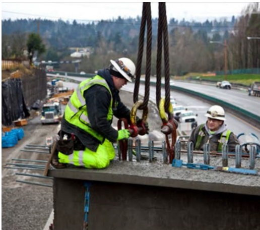
(a) PC girder being lifted using lifting loops
