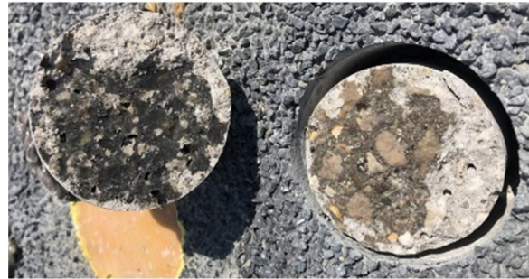
c) E2 epoxy overlay under outdoor summer exposure
