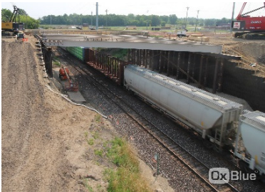
(a) During the construction of replacement superstructure
