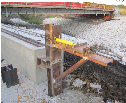
(b) Prestressing jack mounted against a reaction frame (Hawash and Nelson 2014)
