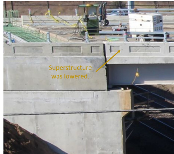
(d) Superstructure on permanent bearings at its final alignment
