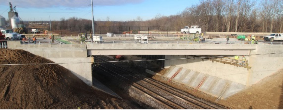
(a) Replacement bridge
