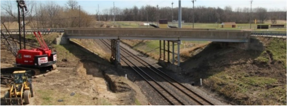
(a) Existing bridge
