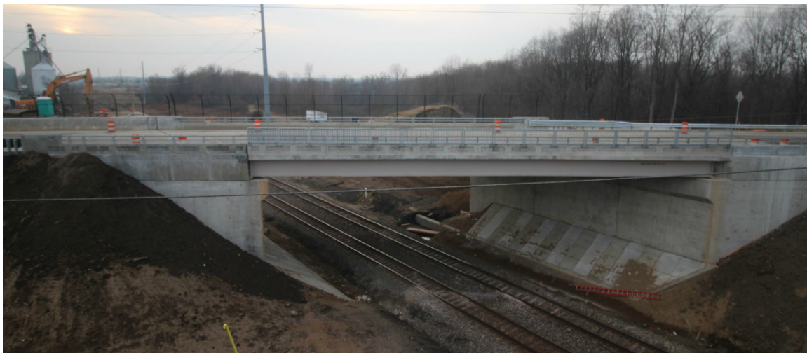
Figure 5-14. View of M-100 over CN railroad bridge site as of December 8, 2015
