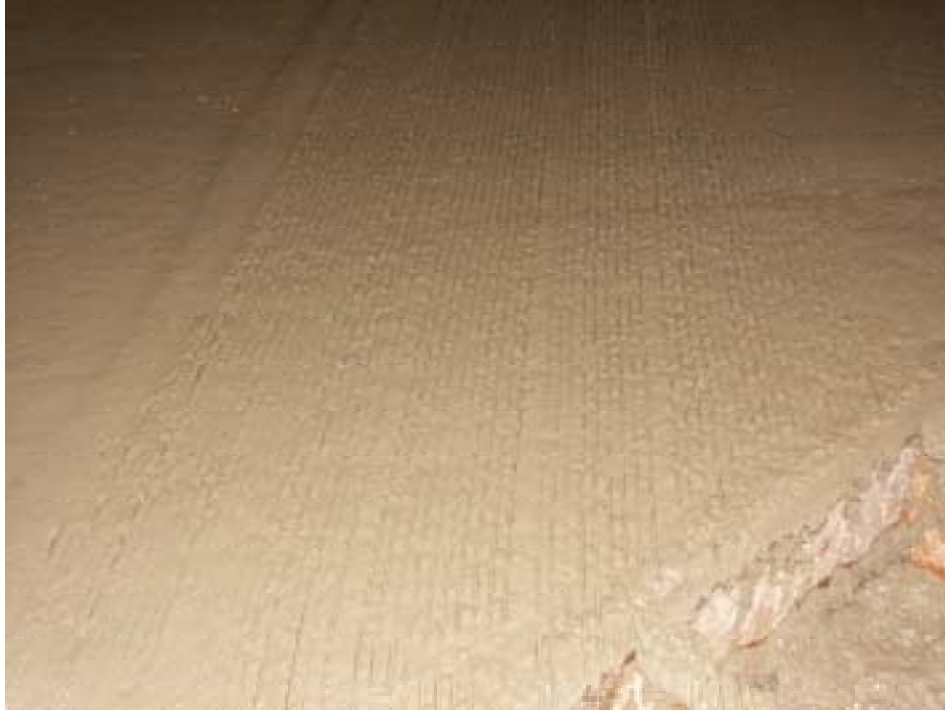
Photo 5-7. Close-up of textured concrete of I-75 over Fort Street
