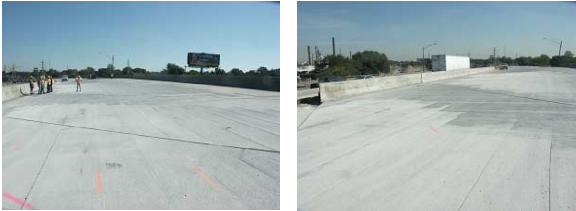
Photo 5-10. Replaced deck of bridge S06 of 82194
