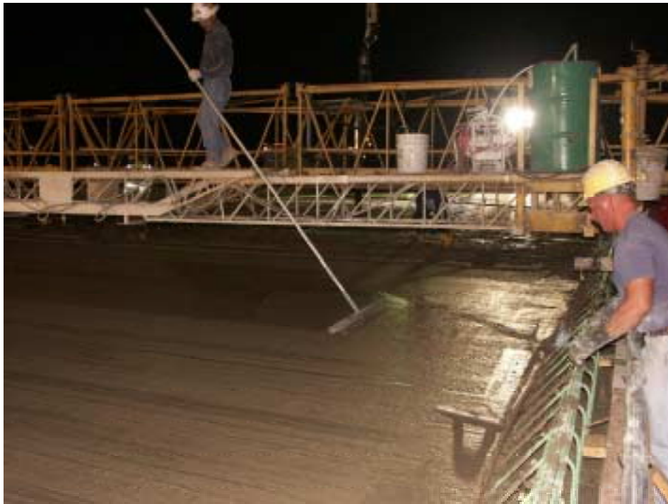
Photo 5-6. Texturing of concrete of I-75 over Fort Street
