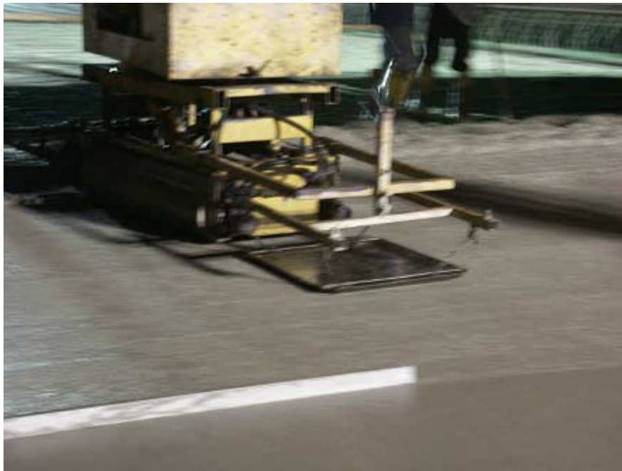
Photo 5-5. Finishing concrete of Vreeland over I-75
