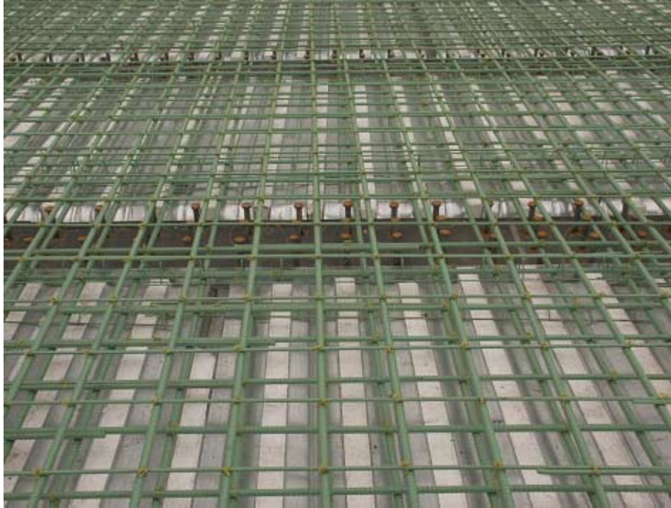
Photo 5-1. Deck reinforcement of I-75 over Fort Street
