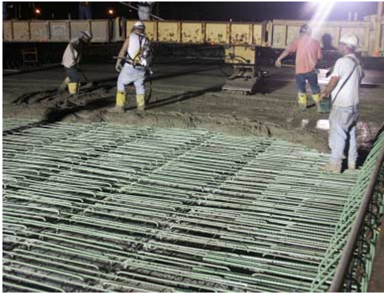
Photo 5-4. Vibration of fresh concrete of Vreeland over I-75
