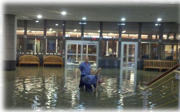
Figure 3-6. Flooding of the Rochester subway (Source: Sederstrom 2013)
