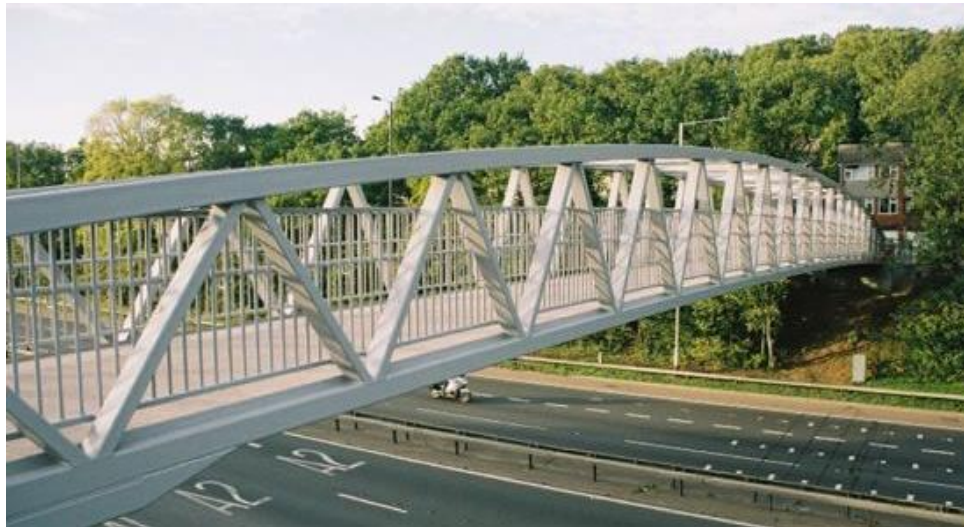
Figure 4-1. A bridge crossing a freeway (Source: Pinterest 2016)
