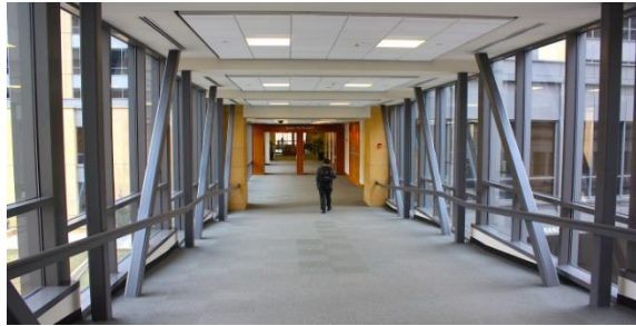
Figure 4-3. An inside view of a skywalk segment in Des Moines (Source: Carole 2013)
