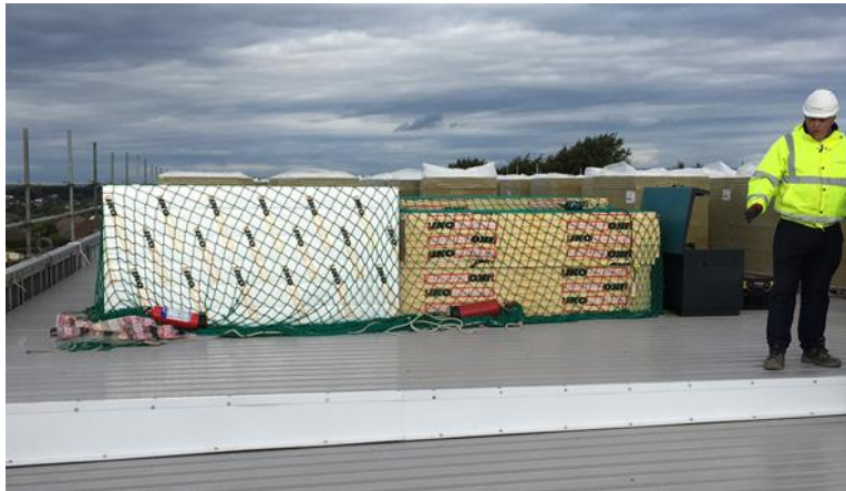
Figure 3-34. Proper storage of roofing materials prior to installation (SIG Design Technology 2014)
