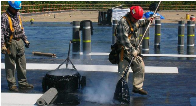
Figure 3-4. Membrane installation using hot asphalt in modified bitumen asphalt roofs - application using hand held mops (Crown Roofing LLC 2016)
