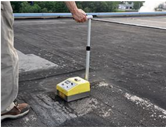
(a) Nuclear scanning meter (Independent Roof Services (IRS) Inc. n.d.)
