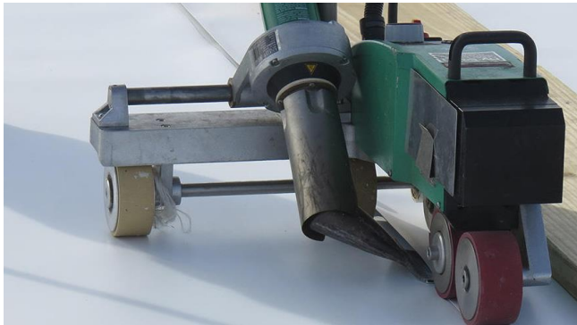
Figure 3-25. Automatic heat welder (Dykstra 2016)
