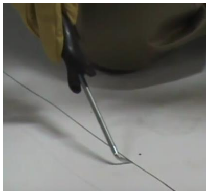
(a) Seam probe testing (Roof Repair 2014)
