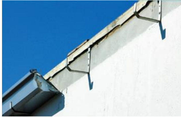
Figure 2-16. Roof gutter with hanger bracket attachment (Smith 2017)
