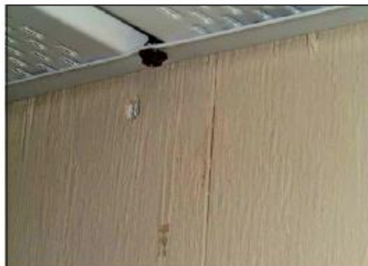
Figure 5. Screws through wall channel.
