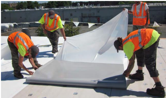
Figure 3-12. Installation of a self-adhered membrane (Sika n.d.)
