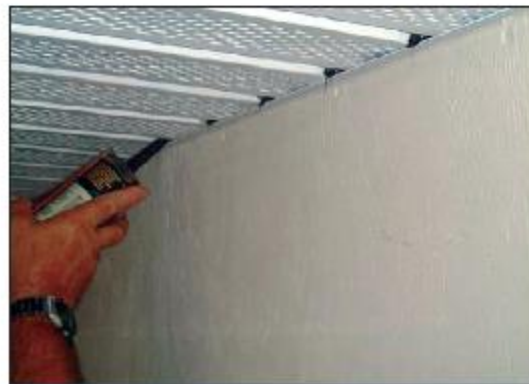
Figure 4. Applying dabs of sealant.
