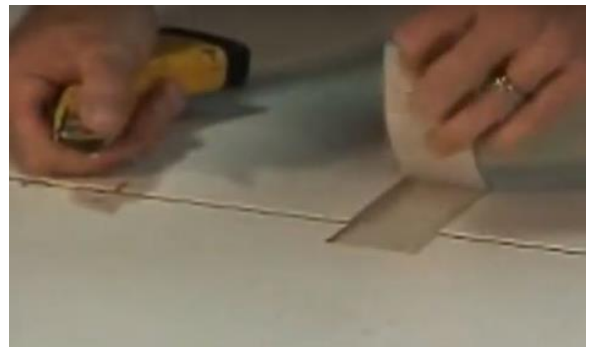
(b) Test cuts – Performing the test cuts (IBRoofSystems1978 2012)
