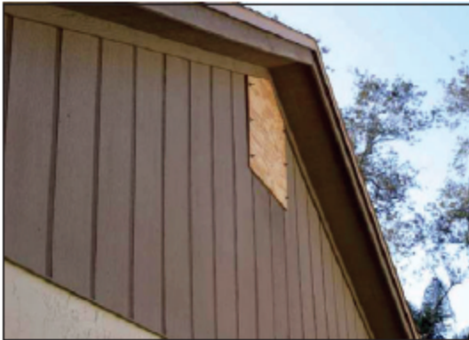
Figure 10. Shuttered gable end vent.
