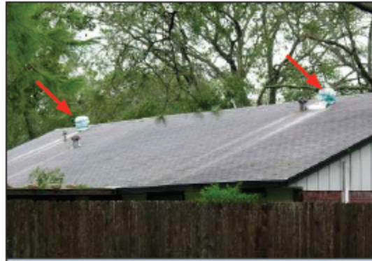
Figure 14. Plastic wrapped turbines.
