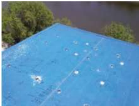
(b) Top surface at the roof corner
