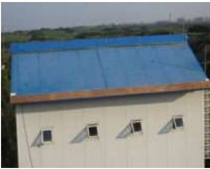
(a) 12 in. (0.3 m) tall parapet along the roof
