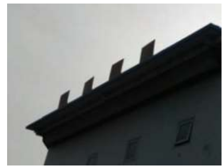
(c) Four segment discrete parapet [one segment is 27.3 in. (0.7 m) tall and 19.5 in. (0.5 m) long]
