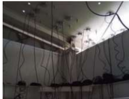
(c) Underneath of the roof corner
