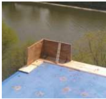
(b) 12 in. (0.3 m) tall and 19.5 in. (0.5 m) long corner parapet
