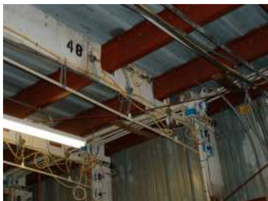
Figure 2-64. Arrangement of pressure measurement tubing and instruments on the roof (Smith et al. 2007)
