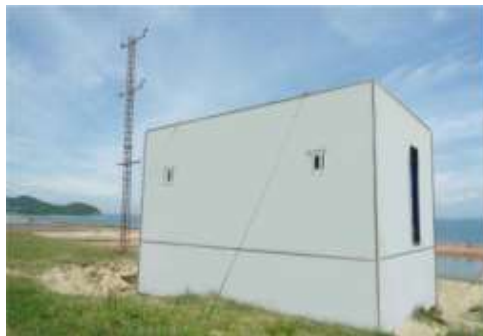
(b) The assembled HNU building
