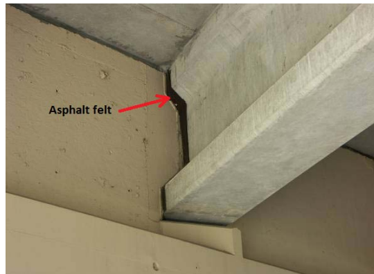
Figure 6-3. Pier-diaphragm-beam end connection details
