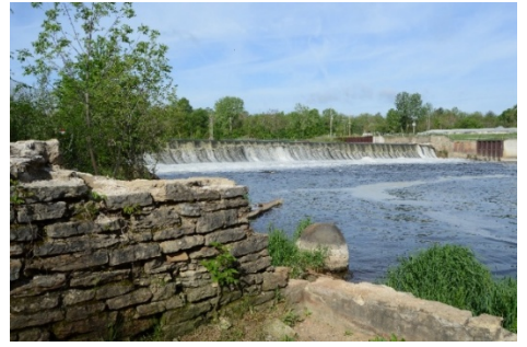
The French Paper Company Dam today.
