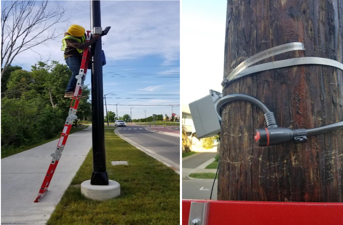
Figure 3.3: Installation of cameras on sites with bike lanes or shared lane markings
